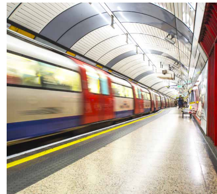
AUTOMATED RAIL MONITORING
